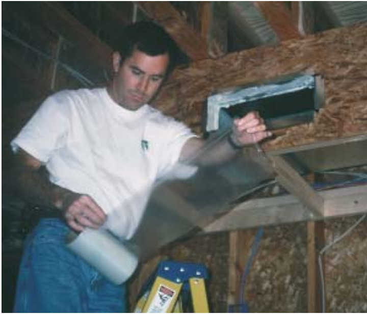
Figure 3. The author carries a roll of adhesive poly Duct Mask on his belt (left) and uses the material to seal registers and grilles (right).
