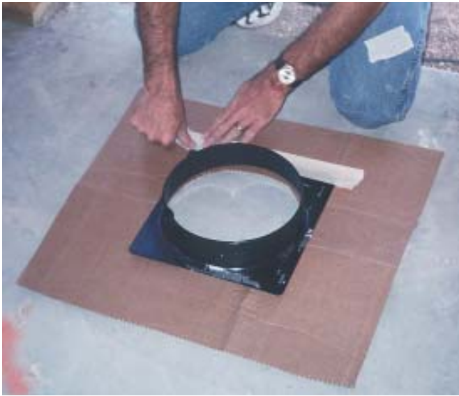
Figure 2. The author tapes a plastic transition fitting to a piece of cardboard cut to fit the opening in the air distribution system (above), then places the assembly in the opening (above right) and connects the fan to the opening with a length of flex duct (right). It's best to test the system with the air handler installed, because the air handlers are often a leakage point. If the air handler has not been set, the author hooks up the Duct Blaster to the trunk line where the air handler will go. The equipment can also be attached to a return grille (below).
