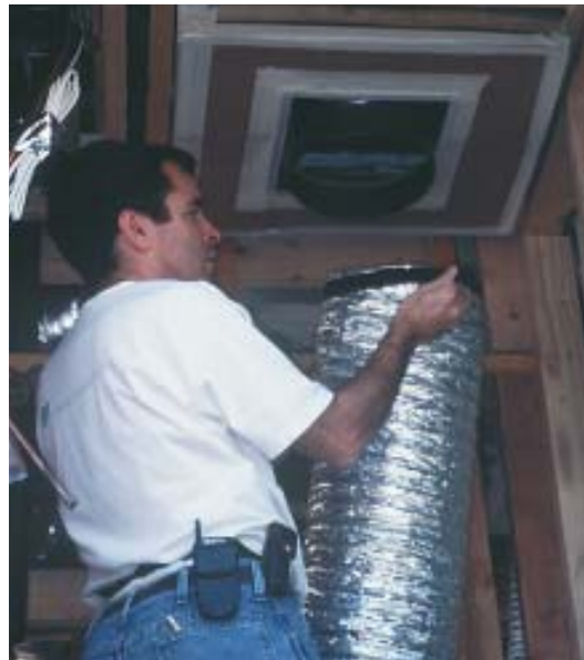
Figure 2. The author tapes a plastic transition fitting to a piece of cardboard cut to fit the opening in the air distribution system (above), then places the assembly in the opening (above right) and connects the fan to the opening with a length of flex duct (right). It's best to test the system with the air handler installed, because the air handlers are often a leakage point. If the air handler has not been set, the author hooks up the Duct Blaster to the trunk line where the air handler will go. The equipment can also be attached to a return grille (below).
