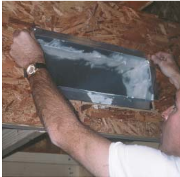
Figure 3. The author carries a roll of adhesive poly Duct Mask on his belt (left) and uses the material to seal registers and grilles (right).
