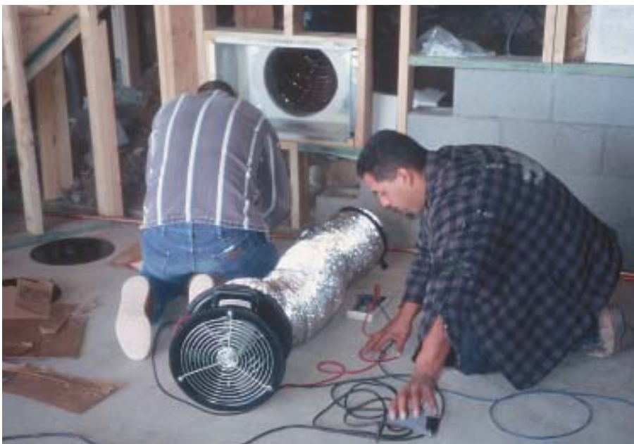
Figure 2. The author tapes a plastic transition fitting to a piece of cardboard cut to fit the opening in the air distribution system (above), then places the assembly in the opening (above right) and connects the fan to the opening with a length of flex duct (right). It's best to test the system with the air handler installed, because the air handlers are often a leakage point. If the air handler has not been set, the author hooks up the Duct Blaster to the trunk line where the air handler will go. The equipment can also be attached to a return grille (below).
