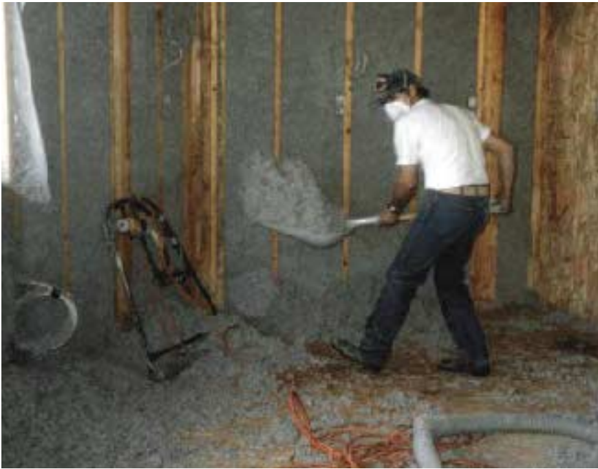
Figure 9. The low-tech method of dealing with excess cellulose is to collect it in clean garbage cans (top) and hand carry it to the hopper (center), where it's mixed with virgin material for reuse (bottom). Newer equipment includes a vacuum system that eliminates most hand work. Either way, it's important to start with a clean, well-swept floor to keep sawdust and other debris from contaminating the insulation.
