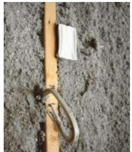
Figure 4. As protection from overspray, windows are covered with poly (left), and electrical boxes are taped over (above).
