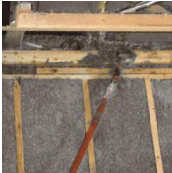
Figure 7. Damp, freshly sprayed cellulose comes off easily, but the material sticks firmly when dry. Corners and other areas too tight for the scrubber to handle are cleaned with a paint scraper fitted with a pole extension.
