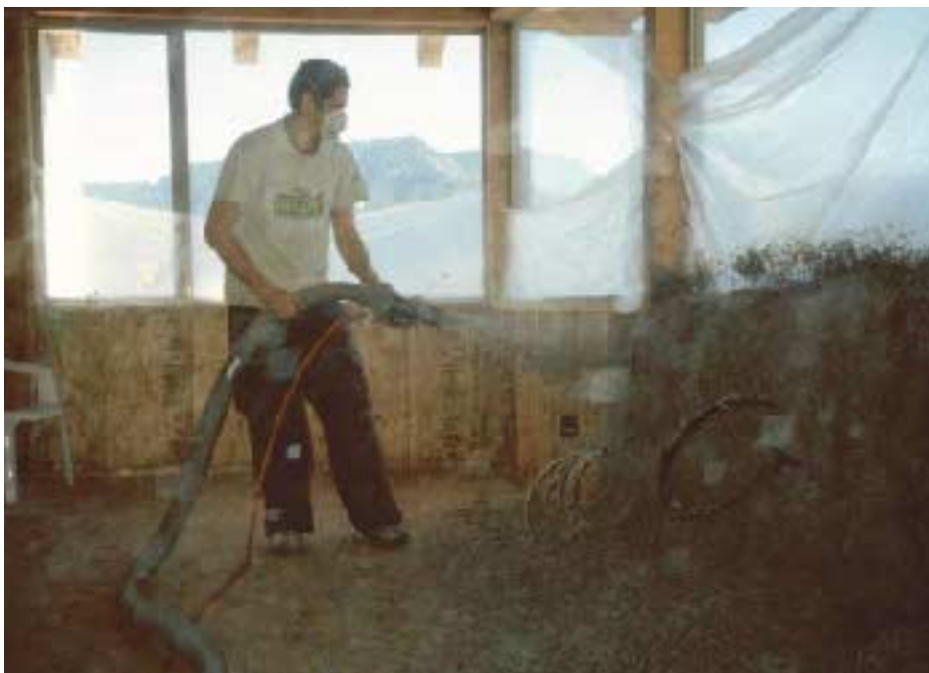
Figure 4. As protection from overspray, windows are covered with poly (left), and electrical boxes are taped over (above).
