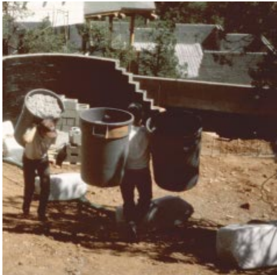
Figure 9. The low-tech method of dealing with excess cellulose is to collect it in clean garbage cans (top) and hand carry it to the hopper (center), where it's mixed with virgin material for reuse (bottom). Newer equipment includes a vacuum system that eliminates most hand work. Either way, it's important to start with a clean, well-swept floor to keep sawdust and other debris from contaminating the insulation.
