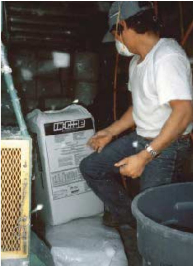
Figure 1. The same cellulose material is used for both wall-spray and loose-fill applications. A typical whole-house wall-spray application requires 60-120 bags.
