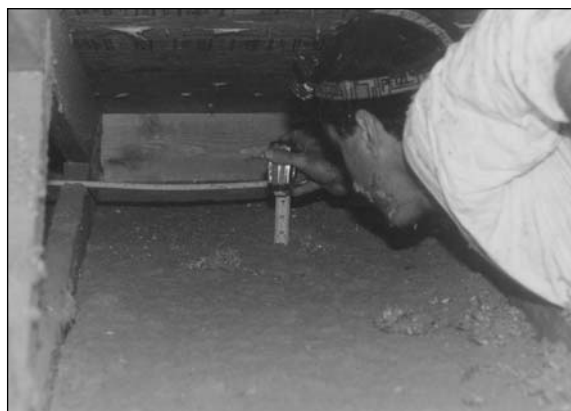
To identify shorting of attic insulation, nothing takes the place of an actual inspection.
