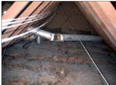
Figure 1. Prime leakage sites include: connections where flex ducts join junction boxes (left), disconnected ductwork (center), and poorly installed boots at grilles and registers (right). Leaky ductwork can spoil the performance of an otherwise tight, well-insulated home.
