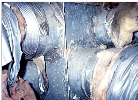
Figure 1. Prime leakage sites include: connections where flex ducts join junction boxes (left), disconnected ductwork (center), and poorly installed boots at grilles and registers (right). Leaky ductwork can spoil the performance of an otherwise tight, well-insulated home.
