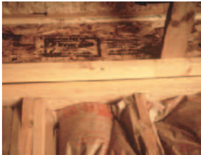
Figure 3. Framers often leave spaces blocked off that are hard or impossible to insulate. Left, the intersection between an interior and an exterior wall can be reached only through a small gap. Above, a wood I-joist has been hung out over the top plate to serve as a nailer for the ceiling drywall, completely blocking access to the band joist. (For the correct detail in this area, see Figure 6.) In both photos, the kraft-faced batts have been jammed into place with no effort to achieve a proper fit.
