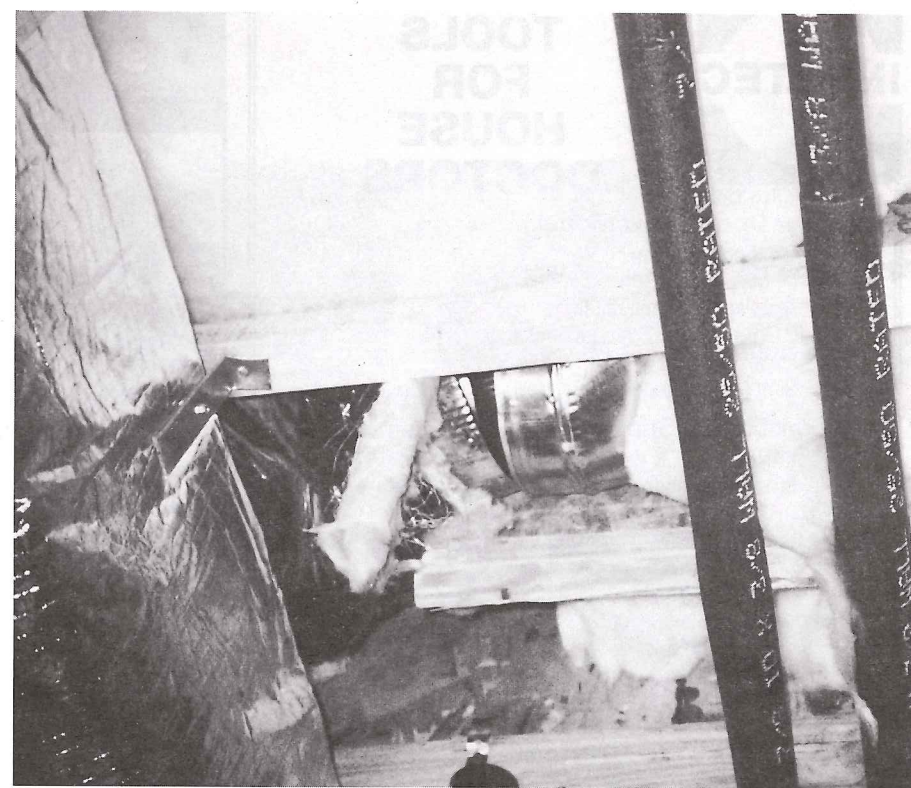
Two obvious energy-wasting problems are evident with this new duct: a disconnection and poor insulation.
